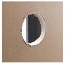
Drill a hole in the drywall with a hole saw AT5 (Ø 74 mm).
